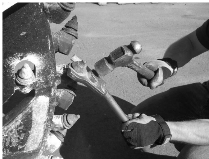
New Pick Installation
